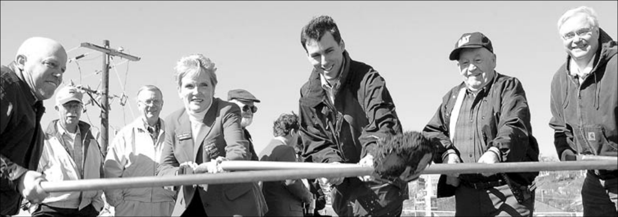
Breaking ground for the Pathway on the Levee are (from left) Duane Grenier, Rotary Club of Galena; Kathy Farlow, Galena Area Chamber of Commerce Ambassadors; Mark Moran, Galena city administrator; Louie Timp, Louie's Trenching; and Scott Lawlor, Galena Grand Excursion. They were joined by 50 others for the festivities. P. Carter Newton photos
